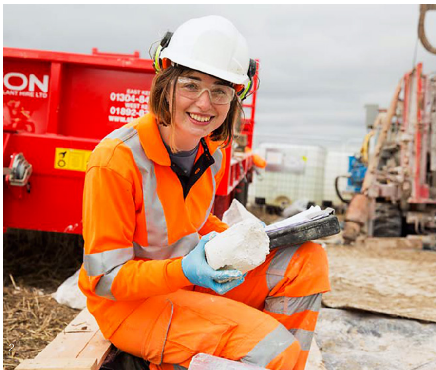
→ Ground investigation works for our A122 Lower Thames Crossing scheme
